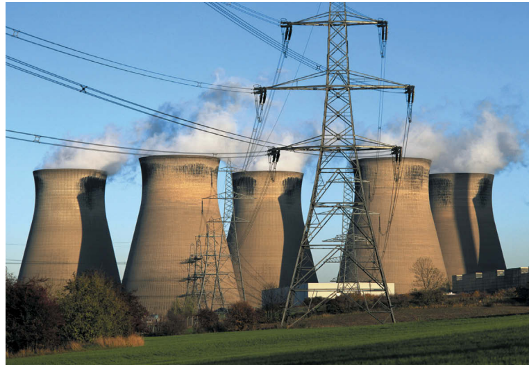
Power project: smart meter plan aims to cost £9.3bn and return £11.8bn over 20 years
